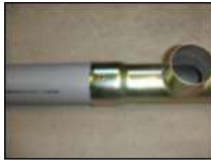
13. The outlet hole on the plastic pipe should be 180 degrees towards the outlet on the T-pipe.
