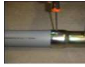
14. Fasten the plastic pipe with enclosed screw.
