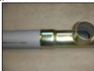
13. The outlet hole on the plastic pipe should be 180 degrees towards the outlet on the T-pipe.
