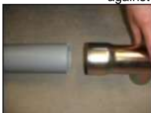
12. Push the plastic pipe together with the T-pipe in the opposite end you drilled the inlet hole in the plastic pipe.
