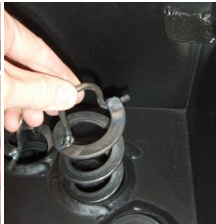
2. Pull up the turbulators appr. 10 -15 cm and drop Repeat a couple of times.
